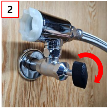
② Turn the water valve to the closed position.
