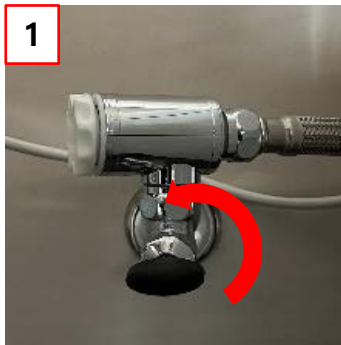
① Turn the water valve fully closed in the direction of the arrow.
