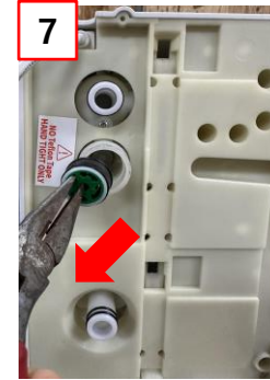
⑦ Pull out the water pressure regulator to remove it.
