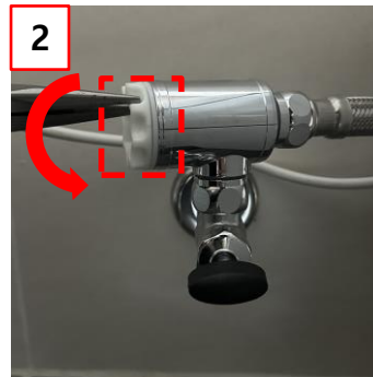
② Use a tool to turn and remove the marked part of the strainer.
