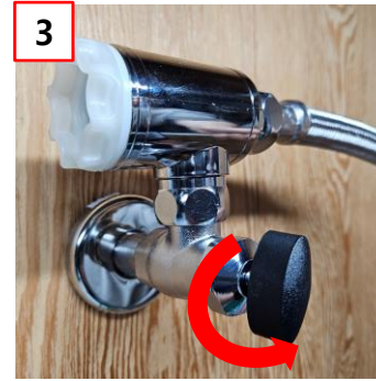
③ Turn the water valve open in the direction of the arrow.
