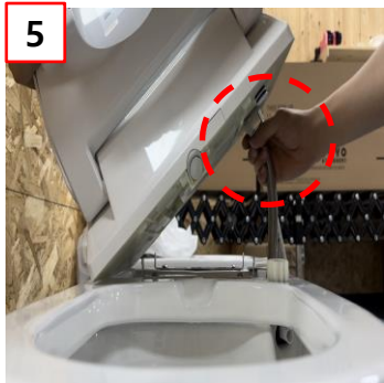
⑤ Disconnect the water supply hose
