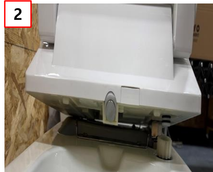
② Align the unit with the base and catch plate, then secure it.
