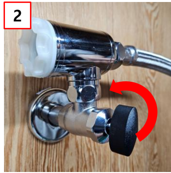
② Turn the water valve fully open in the direction of the arrow.
