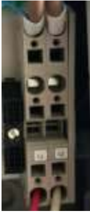
Figure 4.10 AC Connection Area of Inverter
