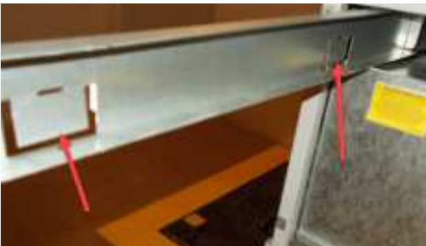
FIGURE 5 Bend Filter Tabs Down
