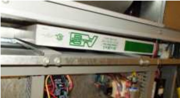
FIGURE 10 Install Left 2" Filter
