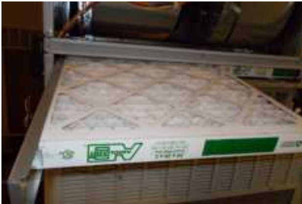
FIGURE 10 Install Left 2" Filter
