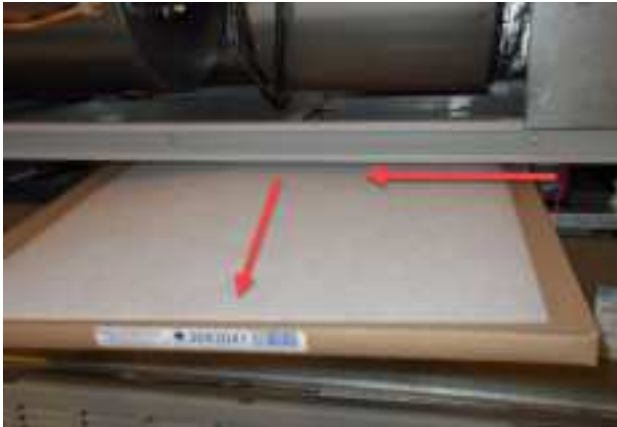
FIGURE 3 Removing Second Filter
