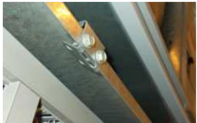
FIGURE 8 Re-Install Screws and Bend Tabs Up
