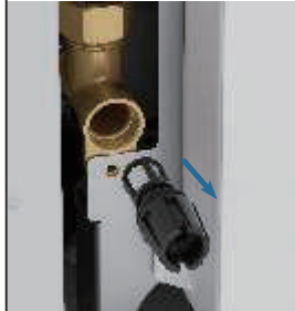
2. Pull out the filter.
